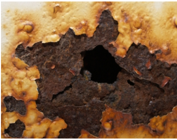
Short lifetime Locker gets corrosive easily as food is hyperhaline
